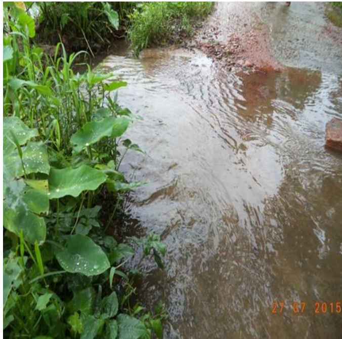
Earthen damaged drain
